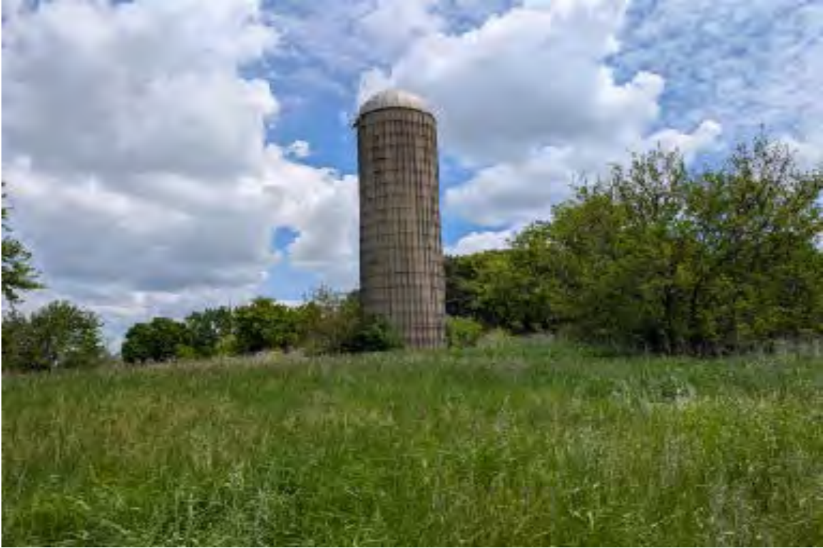
PHOTO 11. View NE of silo in farmstead adjacent to NW corner of Project area (structures off site) (5.27.25)
