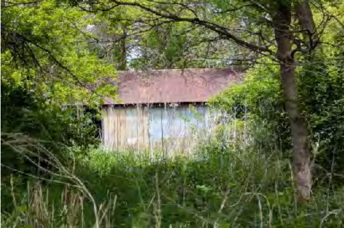
PHOTO 10. View N of structure in farmstead adjacent to NW corner of Project area (structures off site) (5.27.25)
